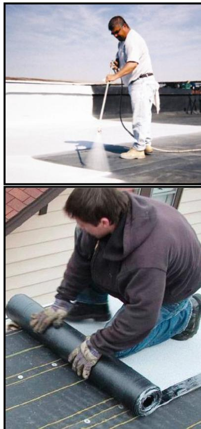
A cool coating is applied to a dark roof (top), and a cool single-ply membrane roof is unrolled (bottom). *Image Source: DIY Advice*
